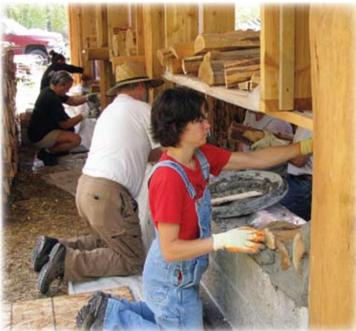
Volunteers laid the cordwood infill on two three-inch-wide mortar beds separated by an insulating layer of dry sawdust mixed with hydrated lime.
