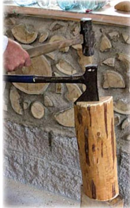
During the infill process, precise sizes and shapes were created using log splitters and hatchets. Volunteers were instructed to make the shapes “funky.”
